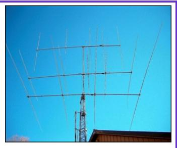
The other two towers (above right and to the right) are 55 foot crankup layovers for HF with monobanders , 10 through 20. The feedlines are LMR600 except for 2m which is 1 5/8 hardline and HF which is some kind of RG8. All the vhf micros are using SSB mast mounted preamps except for 3456 which uses W5LUA preamp by DEMI. Not shown are a 6m, M2 5element yagi , a 6m Ringo and 6m M2 loop on the garage for spotting. The antennas are always a work in progress.
