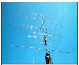
^ On the terrestrial tower: For 6m, two M2 6m7jhv with 15dbd. For 220, one M2 222 7wl with 16.2dbd. For 432, two M2 432-9wl with 20dbd. For 903, one Directive Systems looper 3347lyk with 23.4dbi. For 1296, two Directive Systems loopers 2355lyk with 24dbi. For 2304, one Directive systems 1376ly looper with 23.4 dbi. For 3456, one Directive Systems looper 9112lyk with 25.2d. Micro tower is also a 72ft crankup layover
